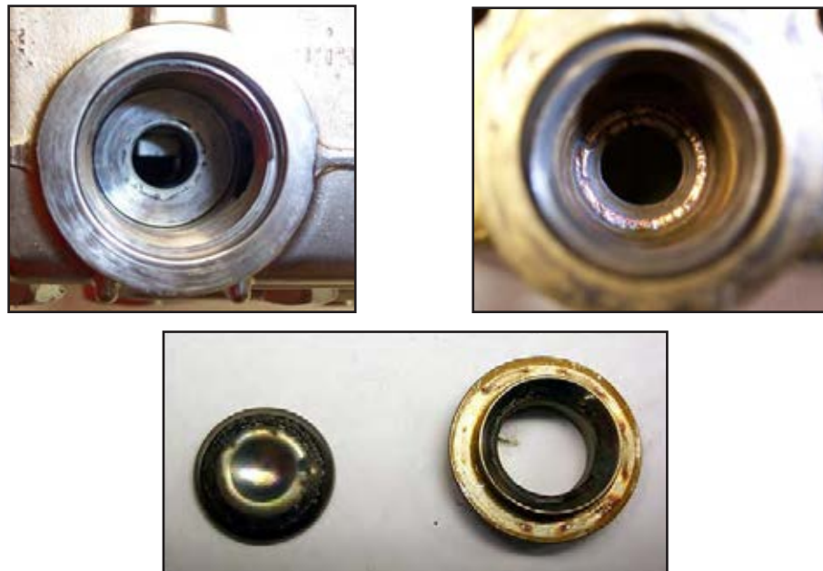
Figure 5-2. Inspect Manifold and Old Valves
